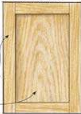
Straight grain on stiles and rails makes for an attractively framed, stable door.
