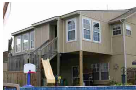
Room Addition to house
